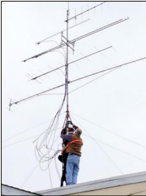
KA3WXV & K3TUF remove rotor and lower mast.
